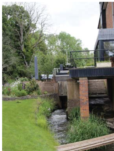
The mill as it is today, running smoothly and putting out about six kilowatthours, even with low water flow.
